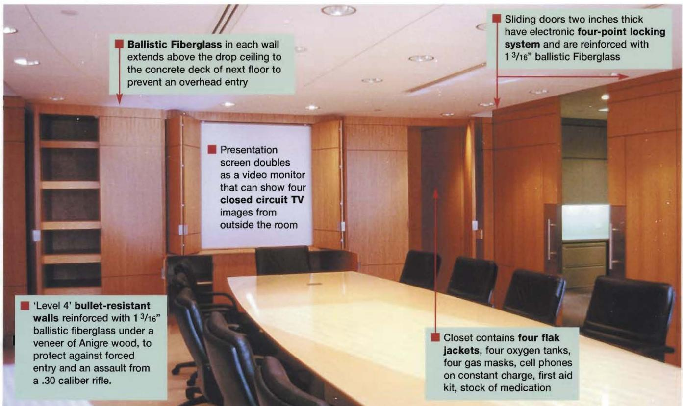
■ **Ballistic Fiberglass** in each wall extends above the drop ceiling to the concrete deck of next floor to prevent an overhead entry
